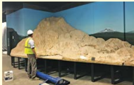
The recently installed Mount St. Helens exhibit awaits painting.
