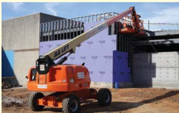
Exterior walls go up around the auditorium.
