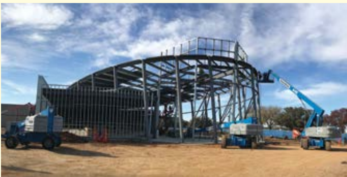
The last steel beams are put in place on the planetarium.
