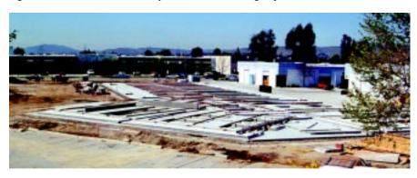
Construction in progress (top). The walls started out horizontal (above). The walls are tilted up, hoisted in place by crane (facing page, left). The last piece of wall goes into place(facing right).
